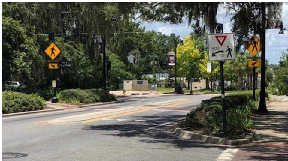
Figure 5.2-4. Pedestrian Crossing Signs (R1-5b and W11-2 with an RRFB)
