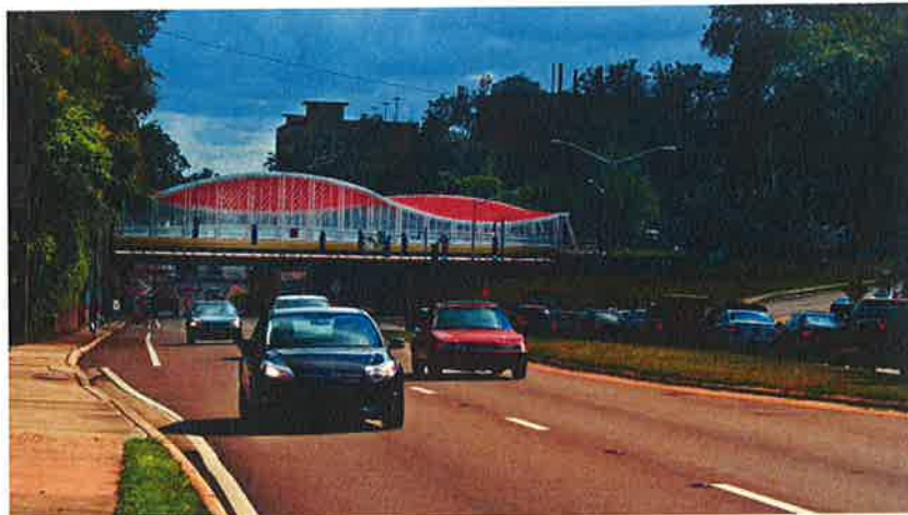
Depot Avenue Rail-Trail Bridge, Gainesville
