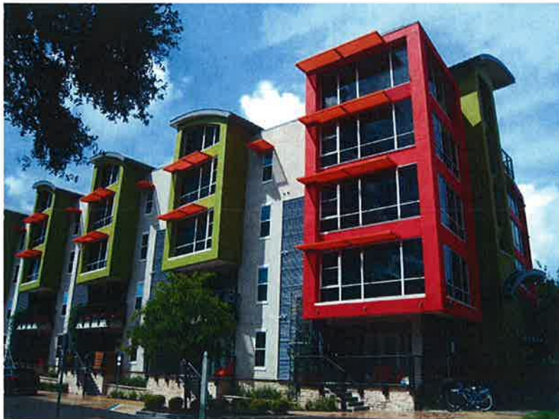
Midtown Redevelopment, Gainesville
