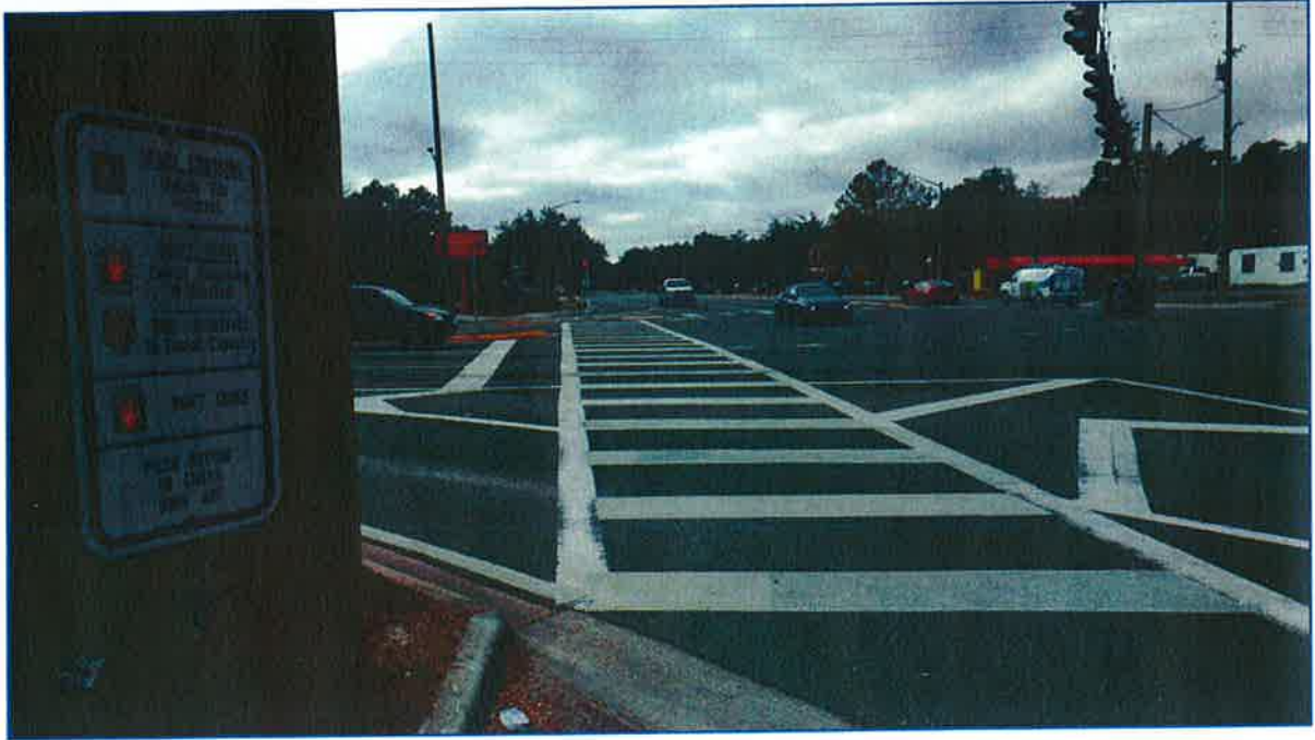
SR 26/SR 24 Intersection – SE Corner looking west
