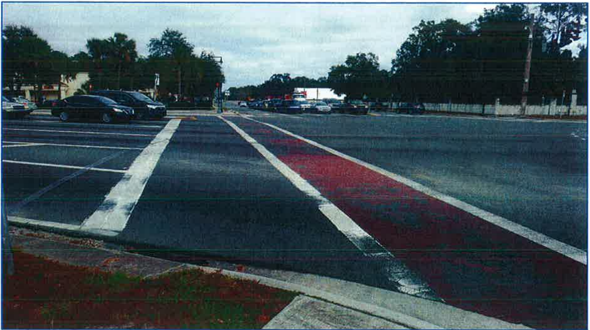
SR 26/SR 24 Intersection - NW Corner looking east
