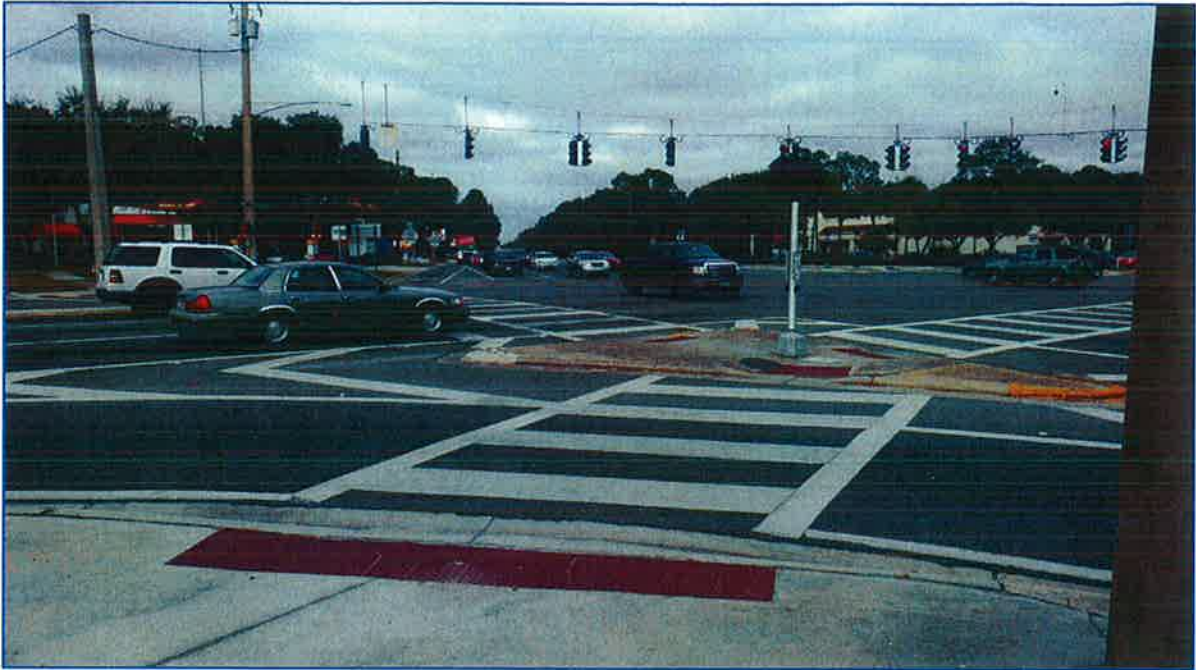
SR 26/SR 24 Intersection - SW Corner looking north
